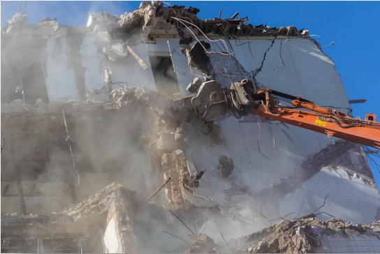
Tear down the wall
